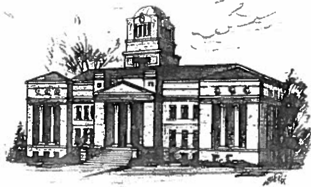
Navarra County Courthouse
