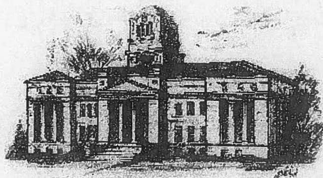
Navajo County Courthouse
